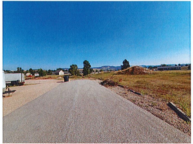
Existing conditions of Ferguson Drive
